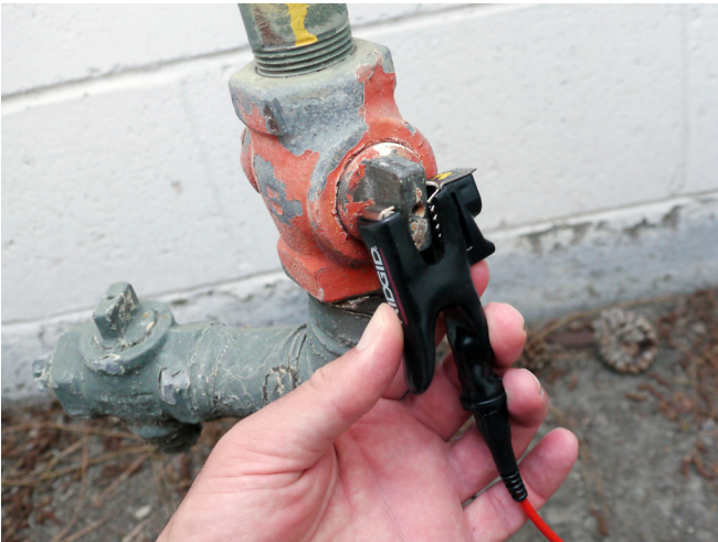
Figure 7 – Connecting the Cable Lead to the Target Conductor
