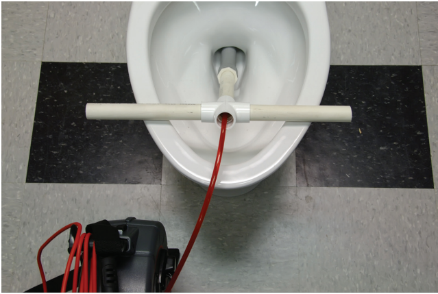
Figure 23 – Using a PVC Guide Tube
