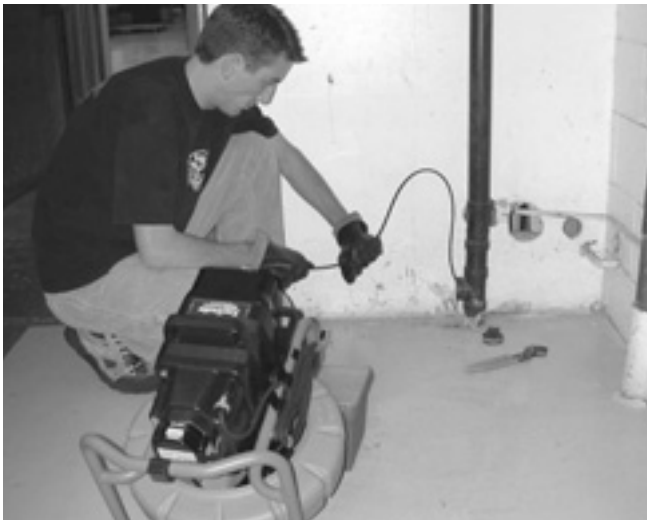
Figure 16 – Incorrect Hand Position on Push Cable
