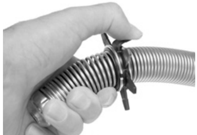
Figure 19 – Pre-stress tabs by placing your finger at the top of the spike and slowly pushing the spike 90 degrees. Repeat in the other direction.
