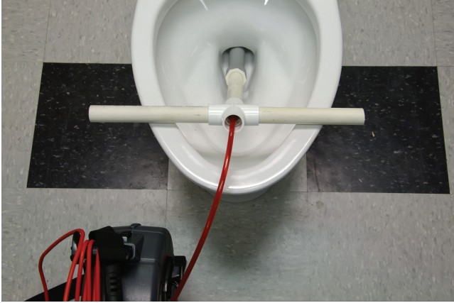
Figure 23 – Using a PVC Guide Tube
