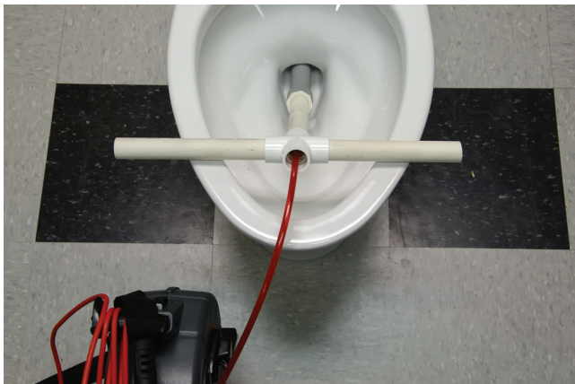
Figure 23 – Using a PVC Guide Tube
