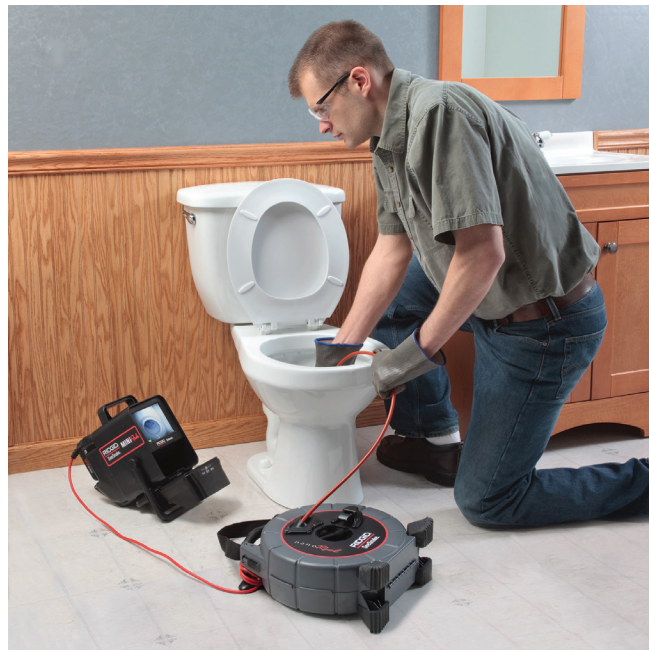
Figure 14 – Performing an Inspection
