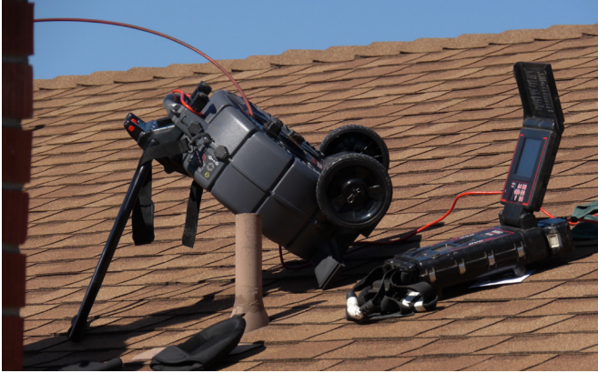
Figure 5 – Positioning for rooftop inspections
