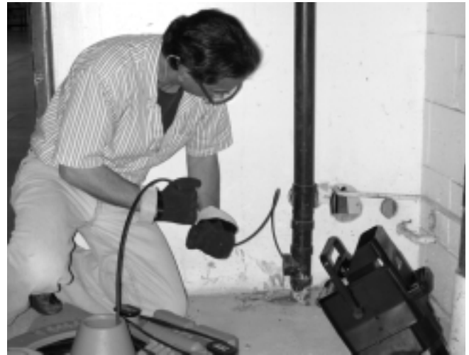
Figure 14 – Incorrect Hand Position on Push Cable
